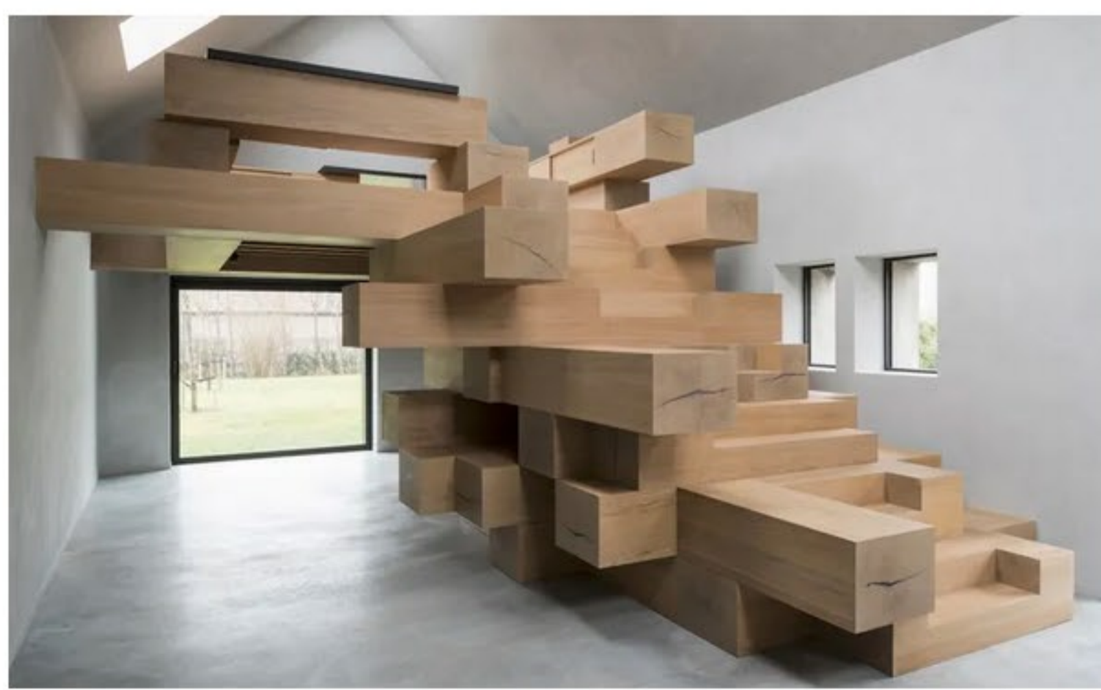
This is achieved thanks to a clever stepped object within, made of thick oak beams connected via steel profiles, which hosts many different uses (Image credit: Koen Van Damme)
