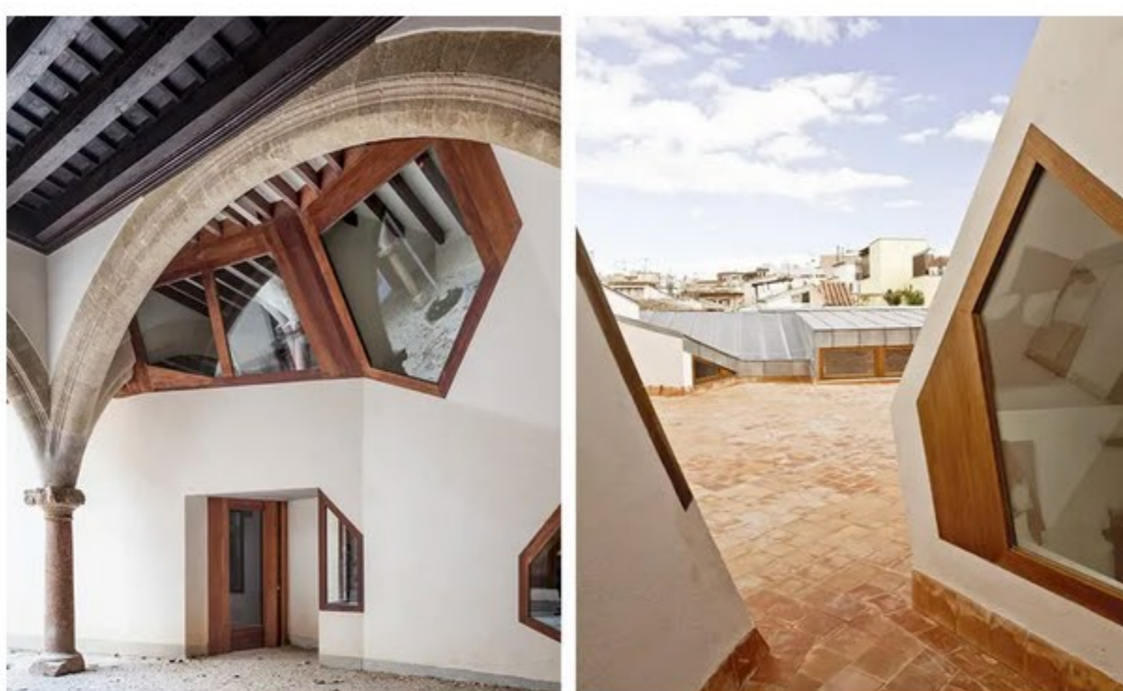
The architects brought plenty of natural light into the building's interiors by creating 'periscopes' set into the roof (Image credit: Adrià Goula)
