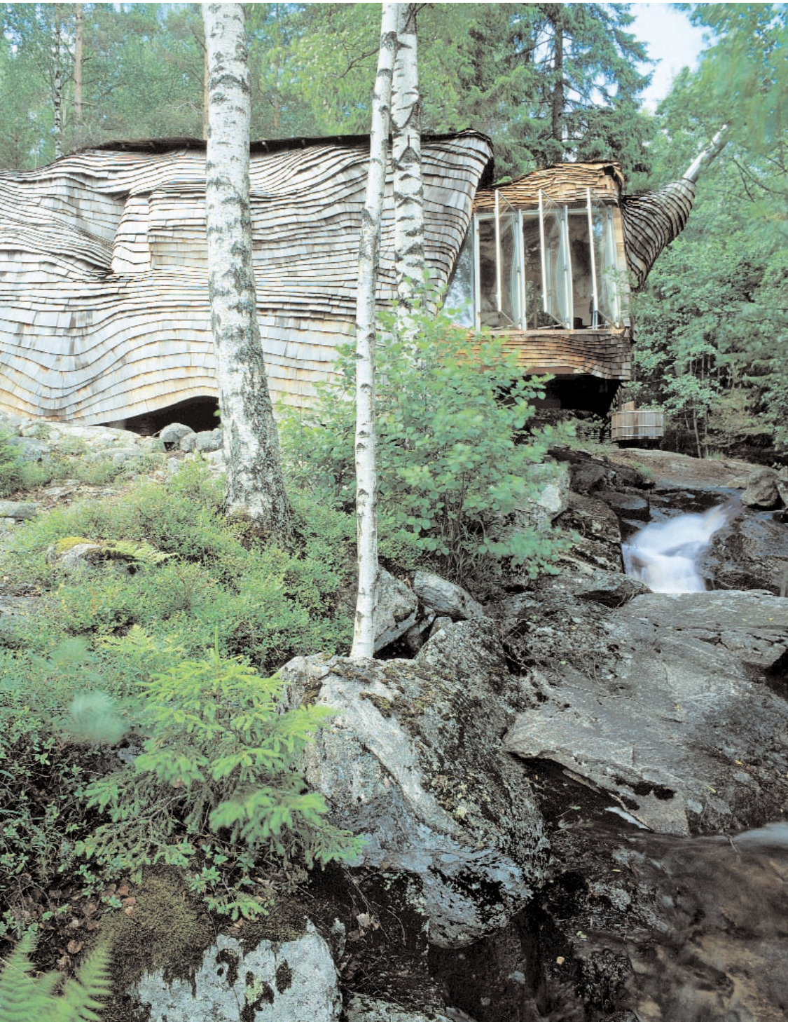
Above: The cantilevered living area, which overhangs the boundary stream, can be retracted manually with a lever-hoist and roller-bearing system.
